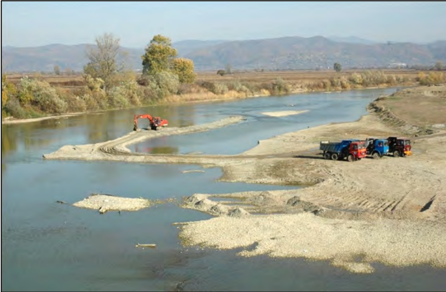
Fig. 13. Alluvial deposits extraction by artificial headlands
