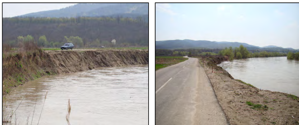
Fig. 10. Shore erosion during the 2010 flood, near Ulmeni
